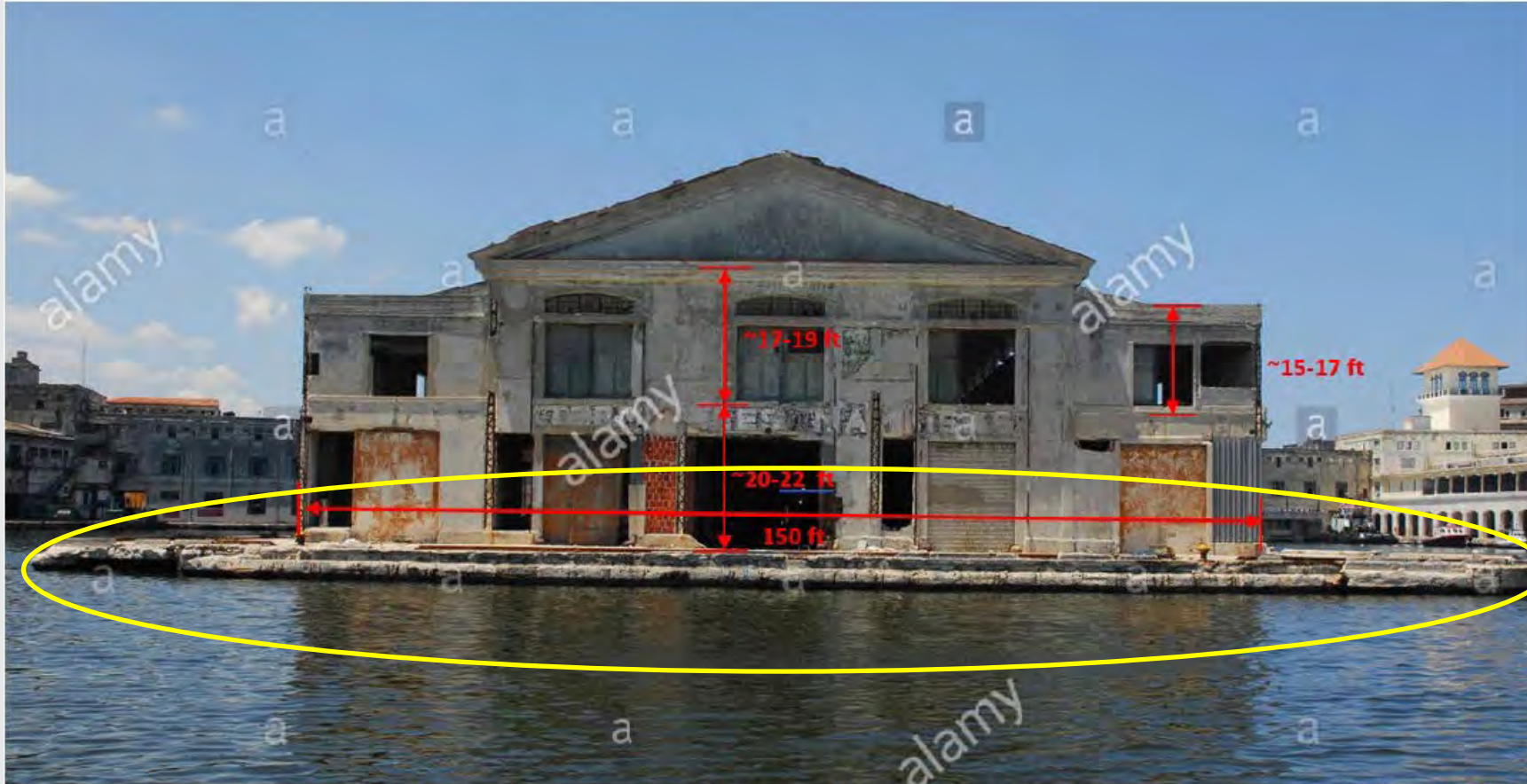
Figure 17 - Estimated Building Dimensions (Alamy - Stock Photos, Stock Images & Vectors 2008), annotated by Collins Engineers, Inc.
