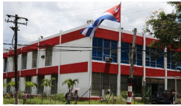
The former Coca-Cola building in Havana, ironically painted the company colors. The Building now houses the headquarters of the state-owned "Beverage Company of Havana". Justin Solomon | CNBC
