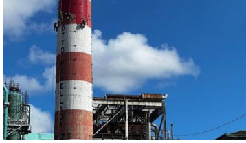
Workers scale one of the smokestacks at the The Otto Parellada Power Plant in Habana. Crédito: Michael Adams
