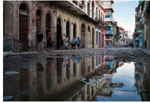
Pedestrians are reflected in the water from a leak in Havana. (Sarah L. Voisin/The Washington Post)
