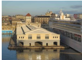
Carnival Corp. is being sued under Title III of the Helms-Burton Act for allegedly trafficking in stolen Cuban property; cruise facilities at Santiago and at Havana, pictured here PHOTO: Anne Kalosh
